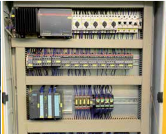
SPS design with signal transfer to superior controls
